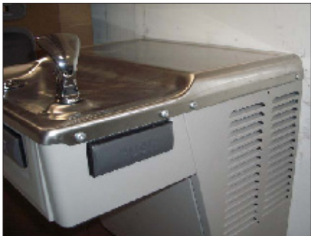
Remove Basin Fasteners
