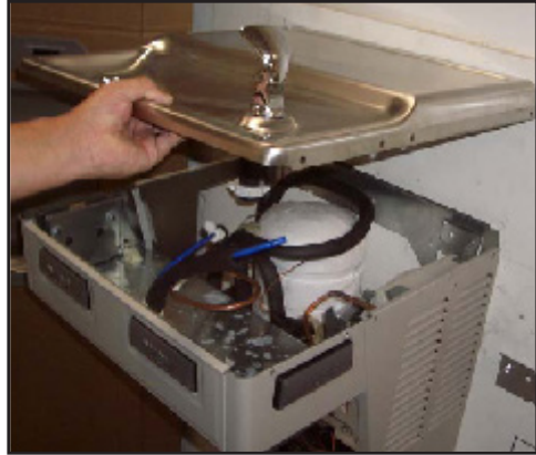
Lift and Remove Basin.
