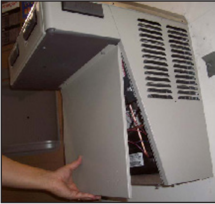
Remove Front Panel
